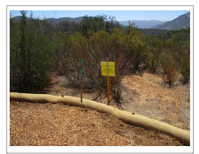
**Photo 2:** During rebar trimming and micropile proof testing at Z571452 (TL6957), an ESA sign was observed along the workspace limits indicating the presence of sensitive status/butterfly host plants (*Plantago erecta*) surrounding the site in accordance with MM BIO-14 and MM BIO-16. Fiber rolls were also observed around the workspace in accordance with the project's SWPPP and ECP (APM HYD-09, MM BIO-7, MM HYD-1).
