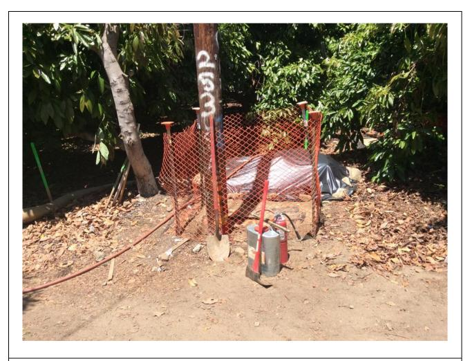
**Photo 6:** The spoils stockpile from the pole hole at Pole P611298 (TL682) was covered with visqueen secured with rocks to prevent erosion in accordance with the ECP and SWPPP (MM HYD-1, MM BIO-7). In addition, the hole was securely covered to prevent wildlife pitfalls, in accordance with MM BIO-23, and a complete set of fire tools was staged on site in accordance with the CFPPP (MM FF-1).
